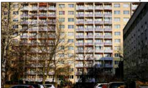
Potsdam, Wohnblock. – Apartment building. Foto: K. Steiof
